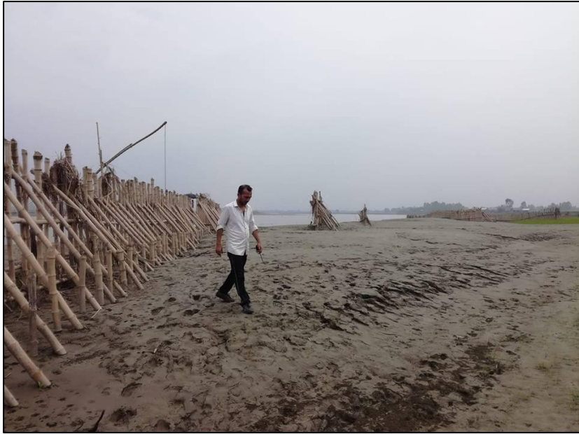
A view of bamboo bandalling for the protection of river bank
